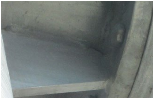
Figure 10-10: Vertical structure connection, missing flat washer on head side of bolt
