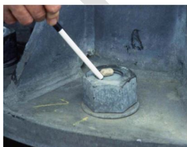
Figure 10-5: Anchor bolts and leveling nuts, anchor nut without fully engaged threads
