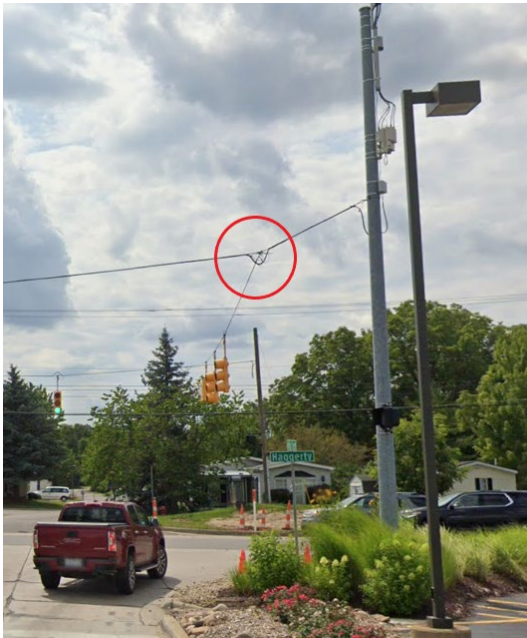
Figure 7-5: Steel strain pole with suspended/hanging box span configuration (suspension circled)
