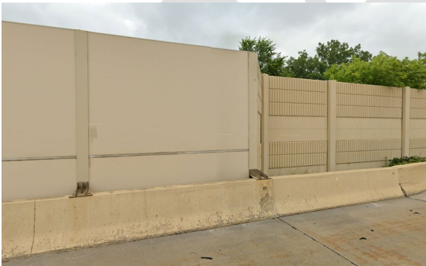
Figure 8-4: Noise wall mounted on crash barrier
