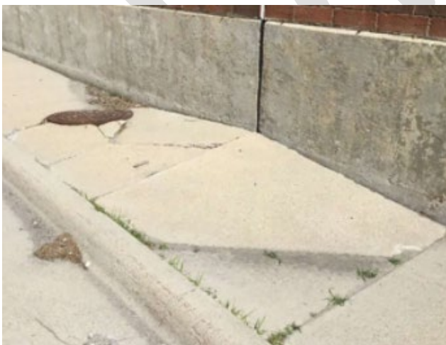
Figure 3-42: Wall settlement
