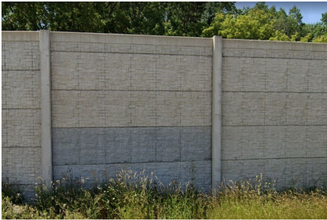
Figure 8-8: Noise wall with vertical joints at posts and horizontal contacts between panels
