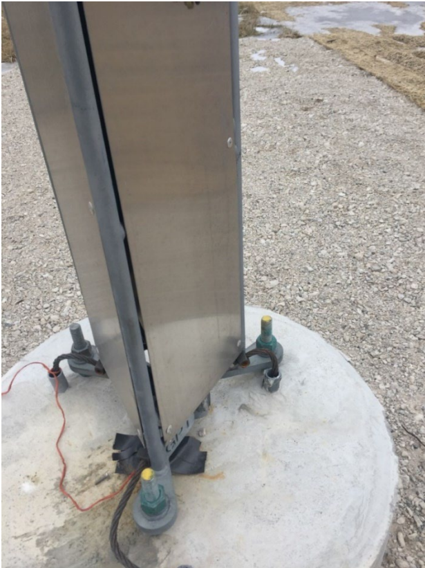
Figure 14-5: ESS tower base plate
