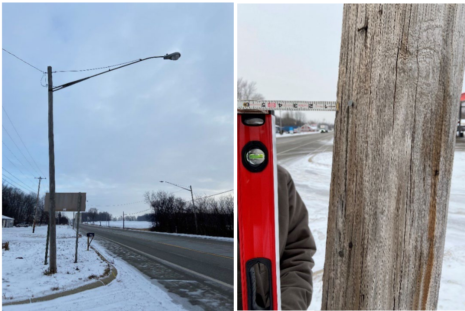
Figure 5-12: Measuring pole misalignment with a 4 ft. level
