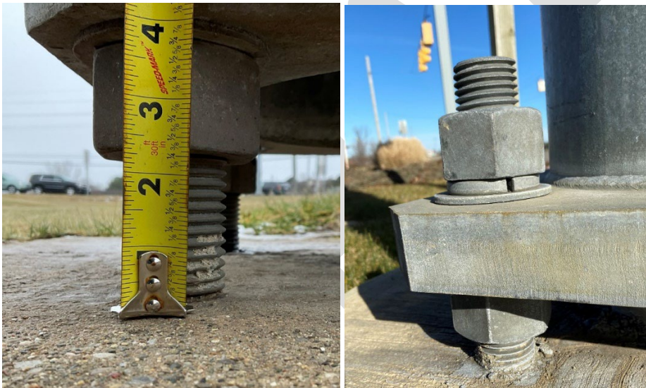
Figure 7-8: Excess anchor bolt standoff distance (left), fully compressed lock washer (right)
