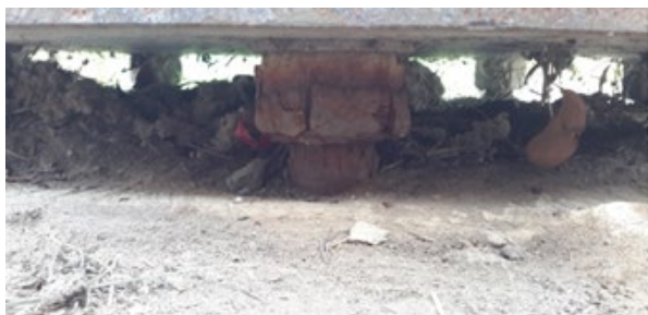
Figure 4-9: Leveling nut and anchor bolt corrosion with section loss
