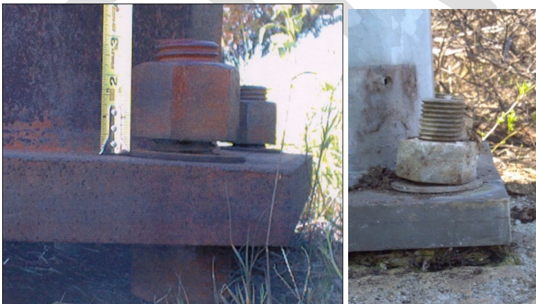
Figure 11-10: Anchor bolt and leveling nut foundation, gap between anchor nut and washer in corroding base unit (left), gap between anchor nut and washer with bolt out of plumb and debris between upright base and concrete foundation (right)
