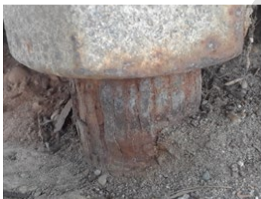
Figure 4-7: Cantilever or truss structure anchor bolts and leveling nuts, corrosion in anchor bolt below upright base with section loss
