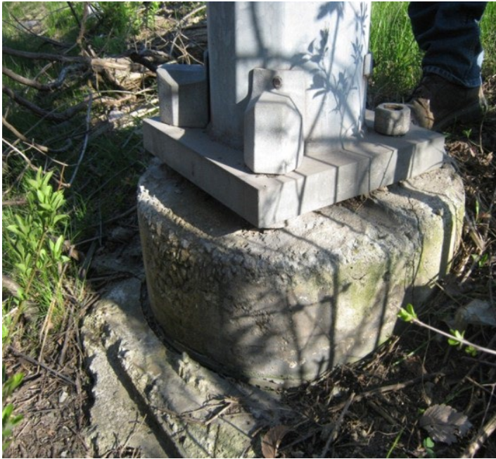
Figure 11-5: Non-frangible concrete foundation deterioration
