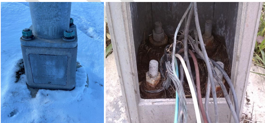
Figure 11-12: Frangible transformer base, panel door present (left), corrosion and debris in transformer base interior with missing panel door, and exposed wires (right)
