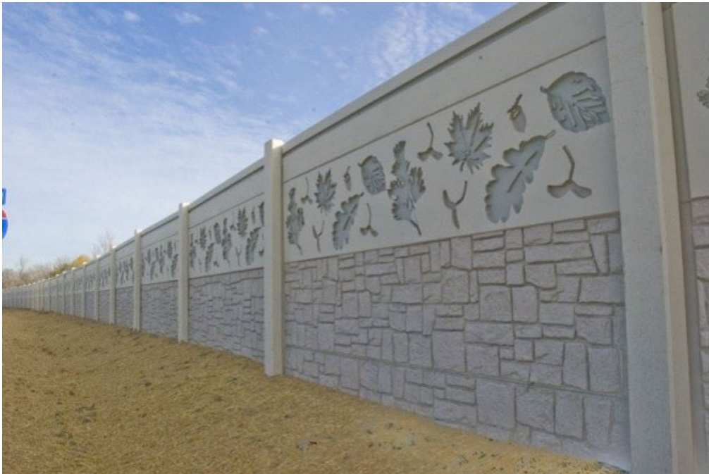
Figure 8-3: Noise wall mounted on soil
