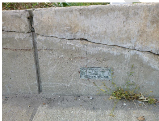
Figure 3-9: Horizontal structural cracking
