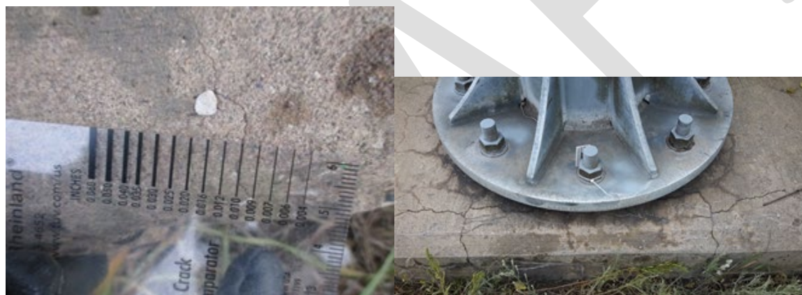
Figure 4-5: Truss or cantilever structure foundation, minor cracking measured with a crack comparator (left), significant cracking (right)
