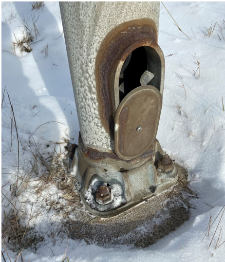
Figure 11-19: Non-frangible pole structure vertical support column (upright), loosely covered handhole
