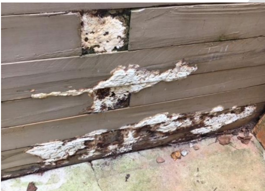
Figure 3-20: Timber lagging splitting
