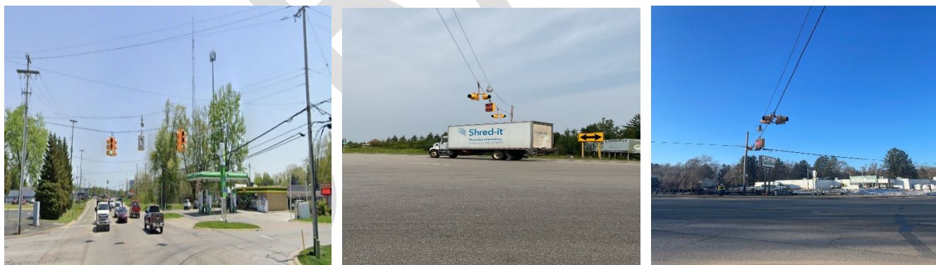
Figure 5-5 Example of Second Span Wire with Luminaire
