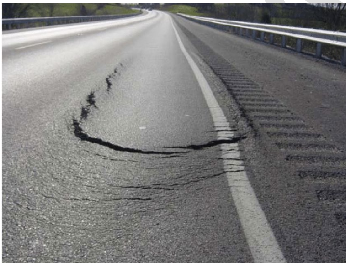
Figure 2-8: Slippage cracking
