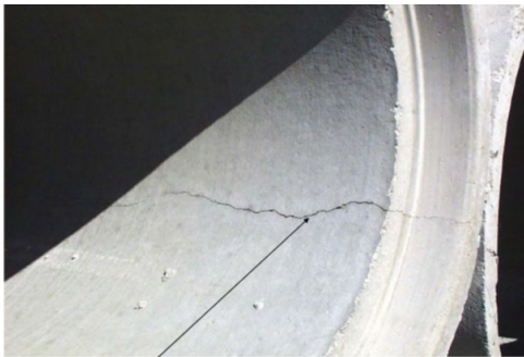
Figure 2-31: Longitudinal crack within a concrete barrel
