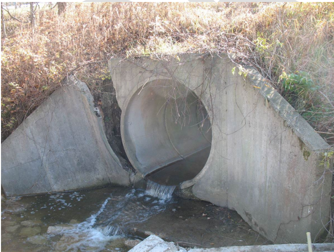
Figure 2-26: Concrete foundation and wingwall damage due to scour
