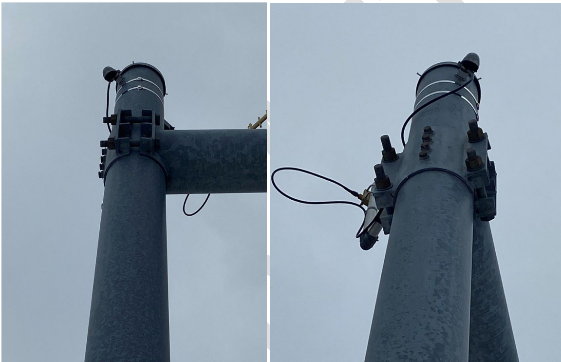
Figure 9-10: Mast arm to pole vertical structure connection, saddle clamp type
