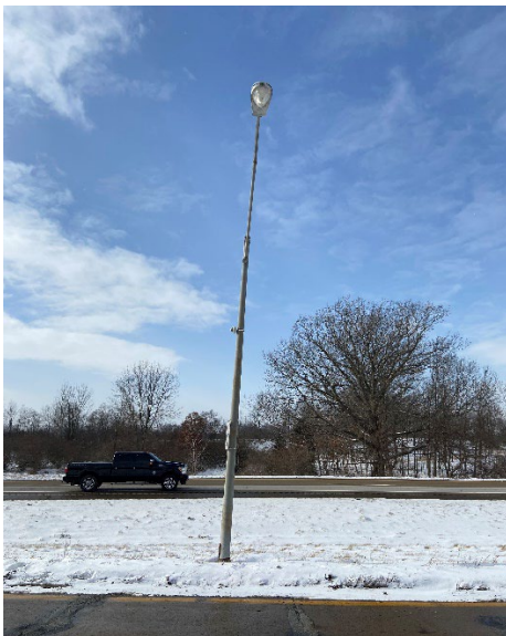
Figure 11-20: Non-frangible pole structure vertical support column (upright), visual identification of out of plumb pole (left), measurement of pole plumbness (right)
