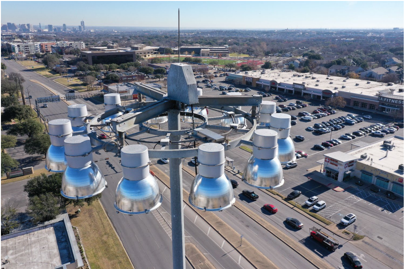
Figure 12-7: HMLT lighting array, as seen from a UAS
