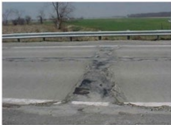
Figure 2-3: Approach roadway, without observable distress (left), clear distress over culvert (right)
