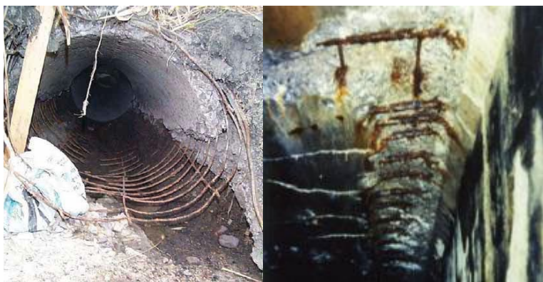
Figure 2-33: Concrete barrel deterioration
