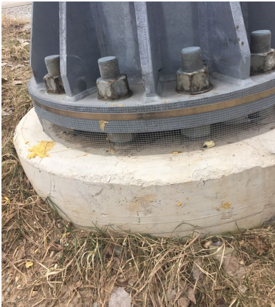
Figure 10-3: DMS support structure foundation, minor spalling
