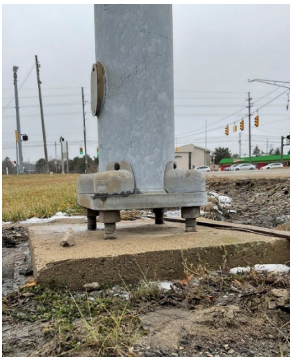
Figure 7-10: Steel strain pole foundation with excess standoff distance and nut covers
