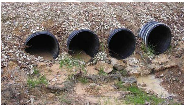
Figure 2-11: Culvert erosion—early-stage gully/rill erosion between the culverts
