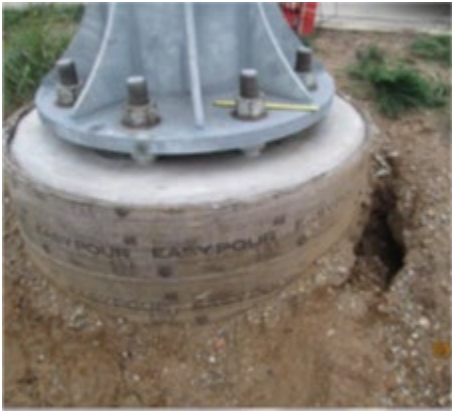
Figure 4-6: Erosion of soil around a truss or cantilever structure foundation
