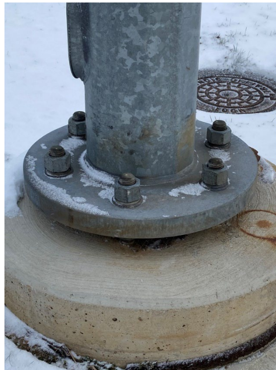
Figure 7-7: Steel strain pole square foundation with four anchor bolts (left, note misalignment), newer style drilled shaft foundation with six anchor bolts (right)
