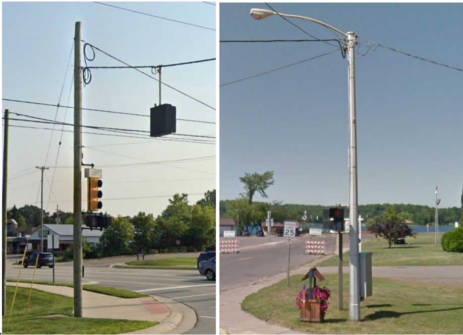
Figure 5-9: Embedded wood pole (left) and embedded steel pole (right)
