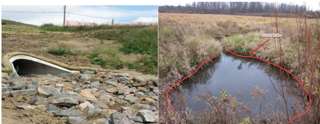
Figure 2-20: No scour (left), scour hole (right)
