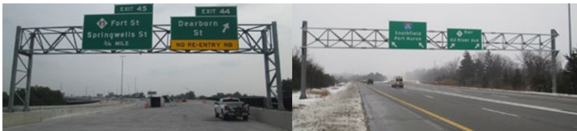
Figure 4-2: Truss structures, box truss (left), tri-chord truss (right)
