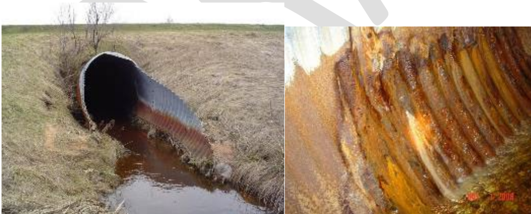
Figure 2-35: Loss of protective coatings contributing to corrosion
