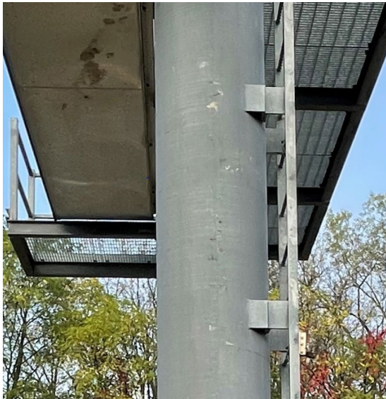
Figure 10-9: Vertical structure column (upright) with minor coating damage
