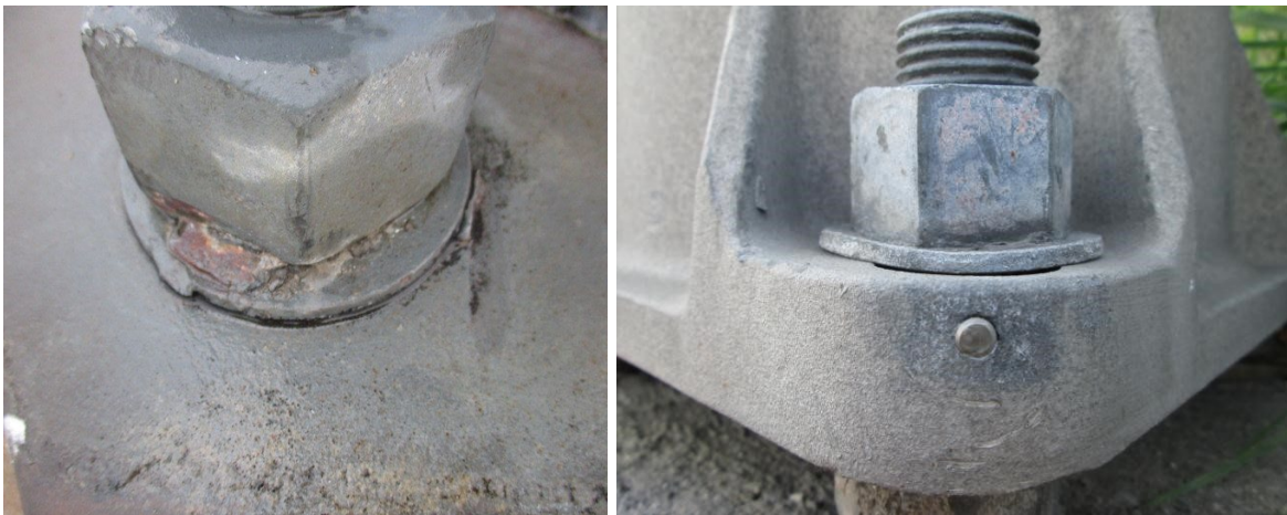
Figure 11-11: Anchor bolt and leveling nuts foundation, nut tack welded to washer (left), incorrect washer type – plate washers intended to cover slotted holes (right)
