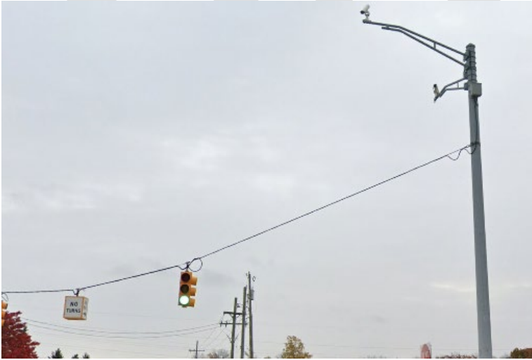
Figure 7-20: Cameras mounted on luminaire truss arms
