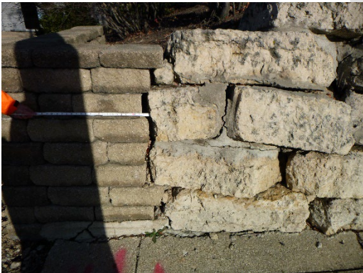
Figure 3-25: Wall misalignment
