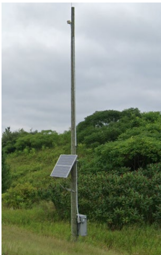
Figure 5-3: Embedded wood pole supporting ITS infrastructure
