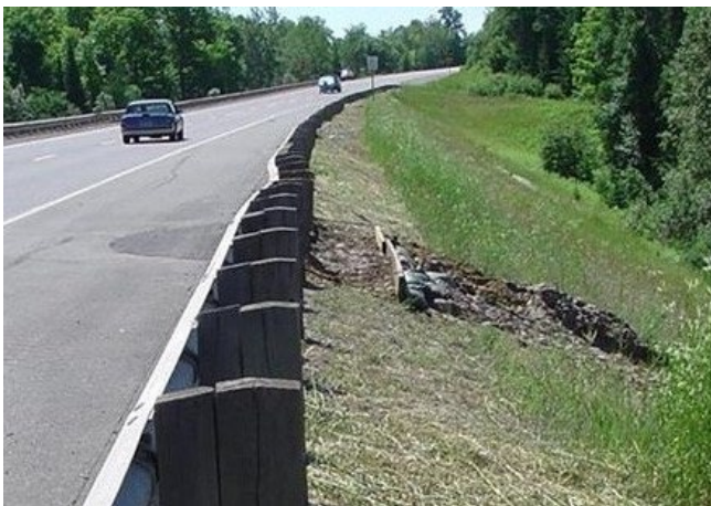
Figure 2-9: Example of embankment failure above a culvert
