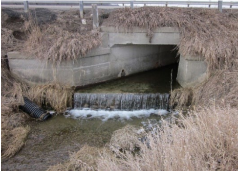
Figure 2-15: Vertical alignment issue leading to stream degradation
