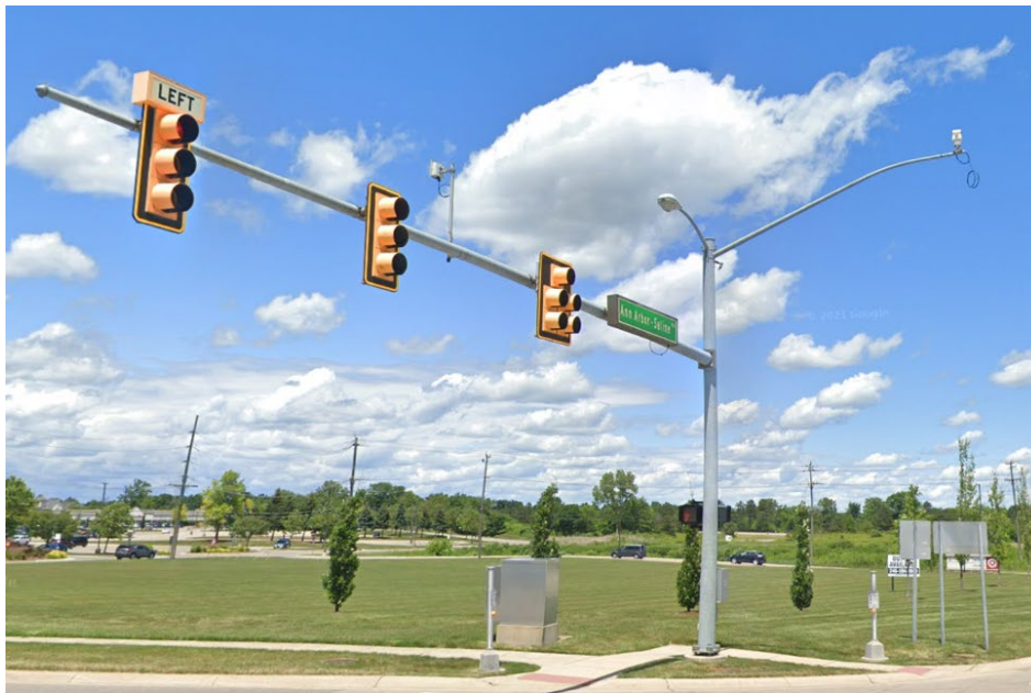
Figure 9-16: Mast arm structure supporting signals, sign, luminaire, camera, and sensor
