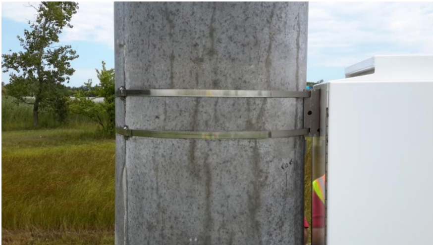
Figure 6-7: Band clamp connection to metal enclosure
