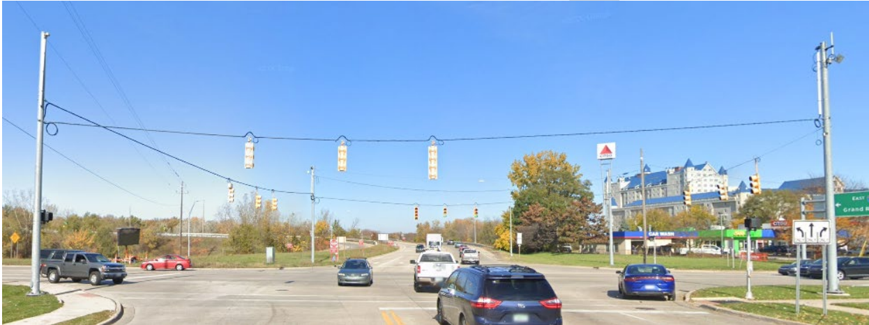
Figure 7-3: Steel strain poles with box span configuration
