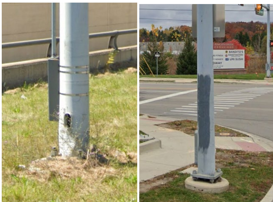
Figure 7-12: Impact damage and missing hand hole cover (left) and graffiti/coatings repair (right)
