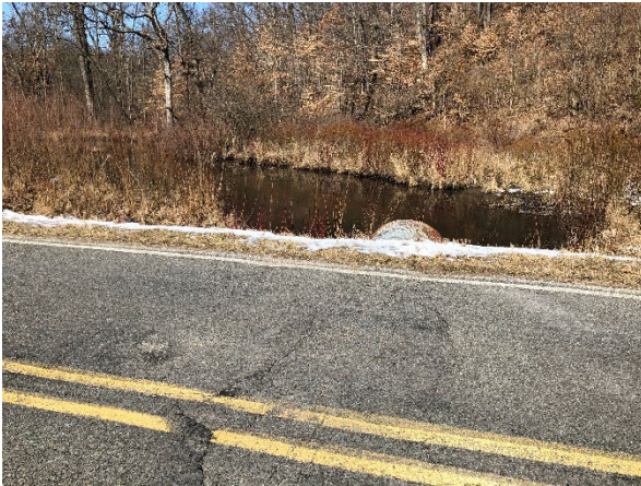
Figure 2-5: Transverse cracking of pavement above culvert
