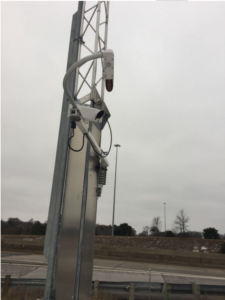
Figure 14-6: ESS tower vertical support column with ITS attachments
