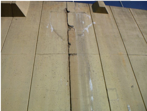
Figure 3-15: Efflorescence accumulation
