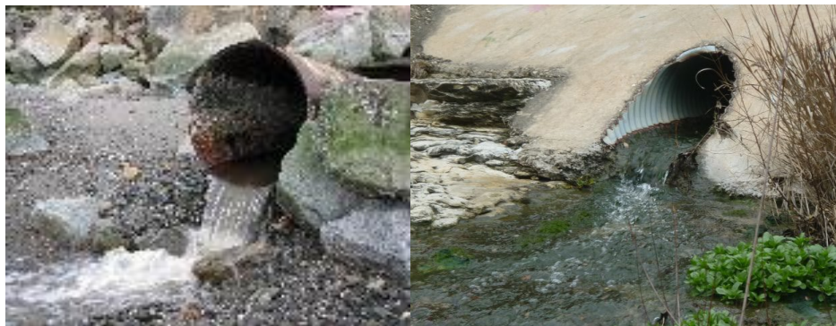
Figure 2-12: Stream channel poor vertical alignment (left) and horizontal alignment (right)
