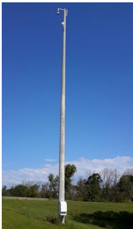
Figure 6-3: Spun Concrete Pole
