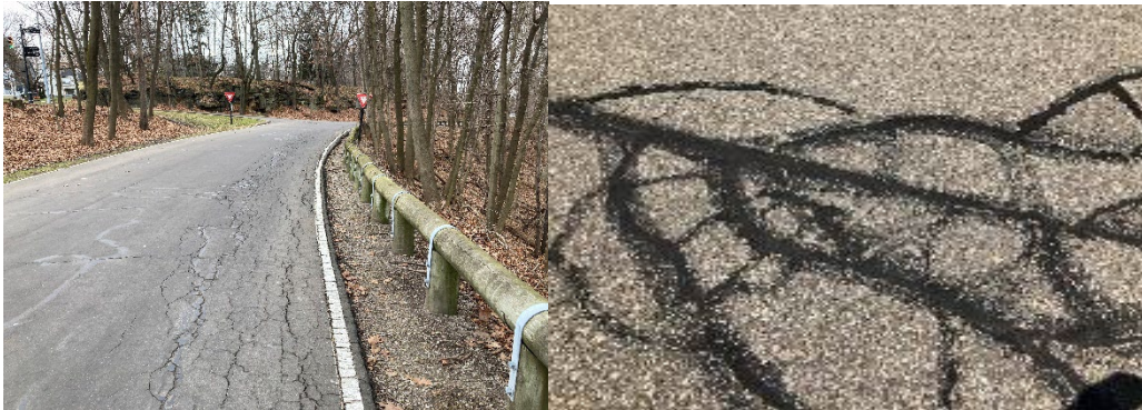
Figure 2-7: Pavement and shoulder alligator cracking
