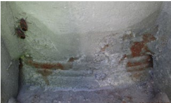
Figure 4-10: Cantilever or truss structure base plate and vertical support, rust underneath galvanizing repair
