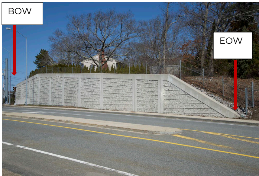
Figure 3-8: Typical wall facing inspection limits
