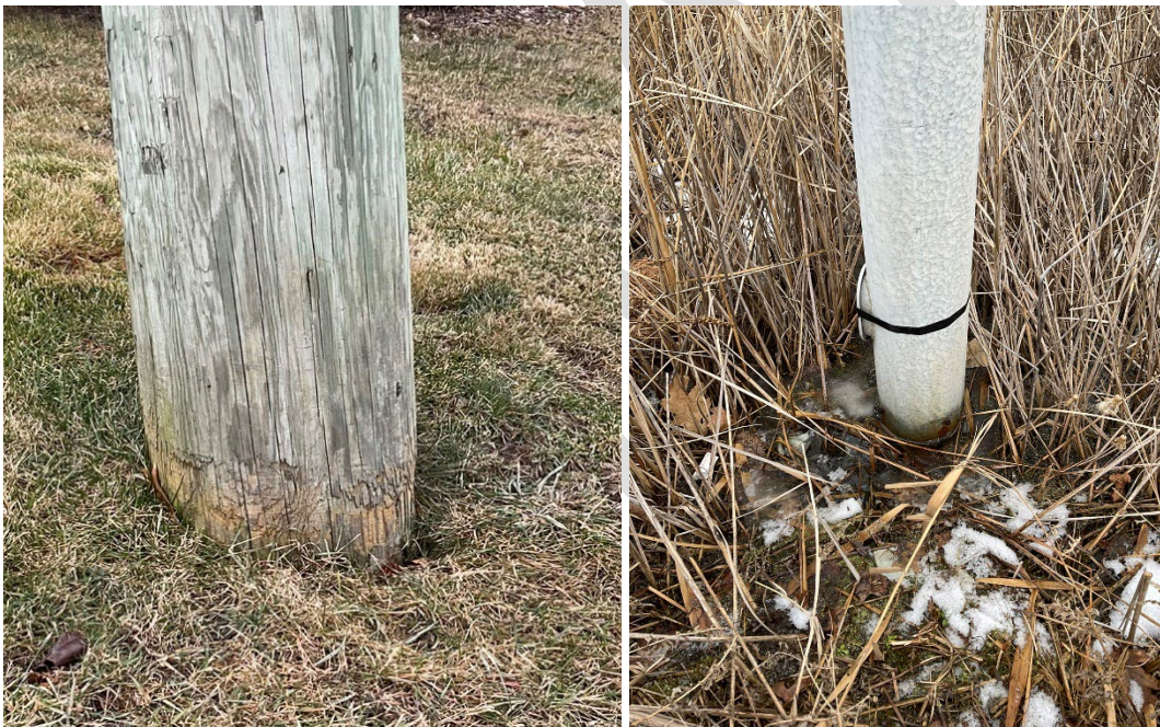
Figure 5-11: Wood pole embedment (left), steel pole embedment (right)
