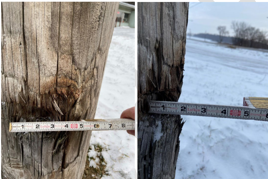
Figure 5-13: Measuring impact damage
