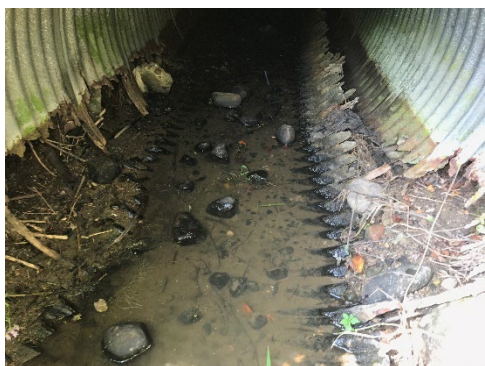
Figure 2-36: Abrasion wearing away corrugated metal pipe corrugations
