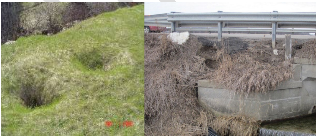
Figure 2-10: Example of embankment issues due to piping (left) or erosion (right)
