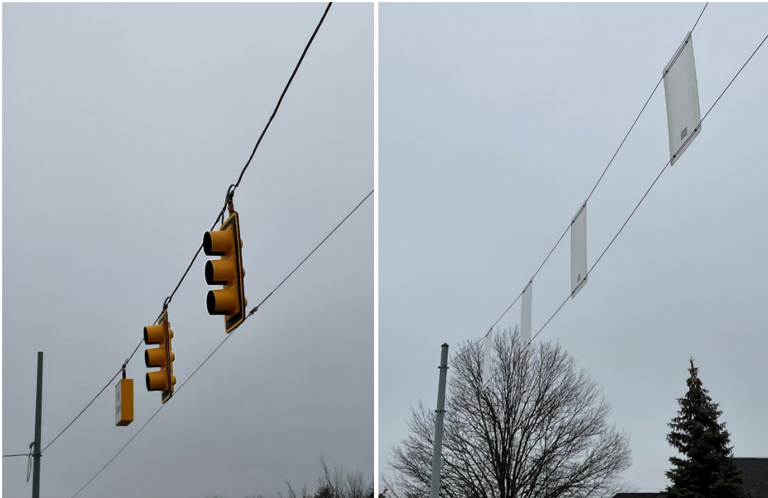
Figure 7-17: Span wire supporting signals and sign (left), span wires supporting signs (right)
