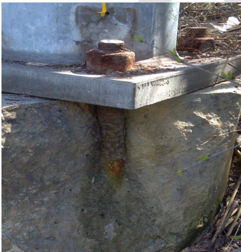
Figure 11-6: Concrete foundation , exposed anchor bolt in damaged foundation
