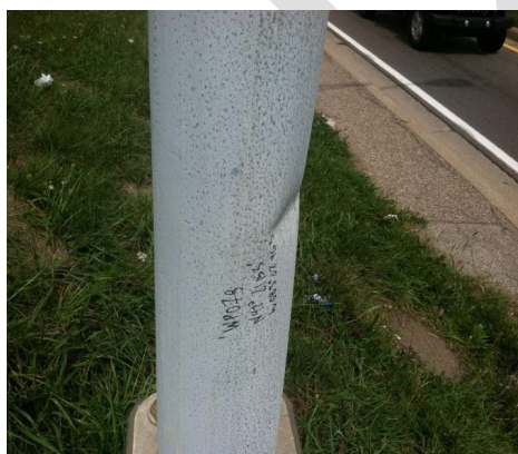
Figure 11-18: Non-frangible pole structure vertical support column (upright), dent
