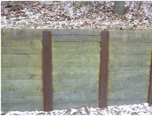
Figure 3-21: Timber lagging is split along top
