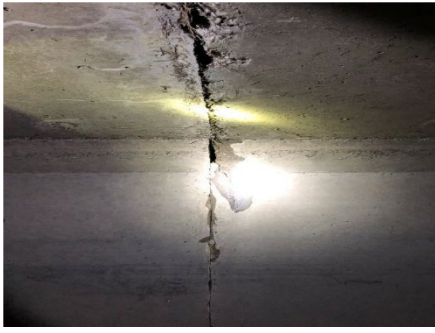
Figure 2-32: Spalling within a box culvert
