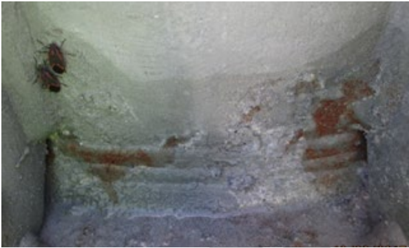
Figure 10-7: Vertical supports, rust underneath galvanizing repair
