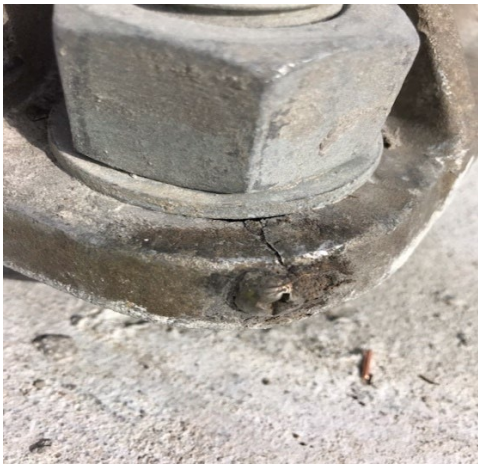
Figure 11-14: Non-frangible pole structure base plate crack
