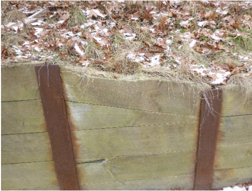
Figure 3-19: Section loss at top of wall
