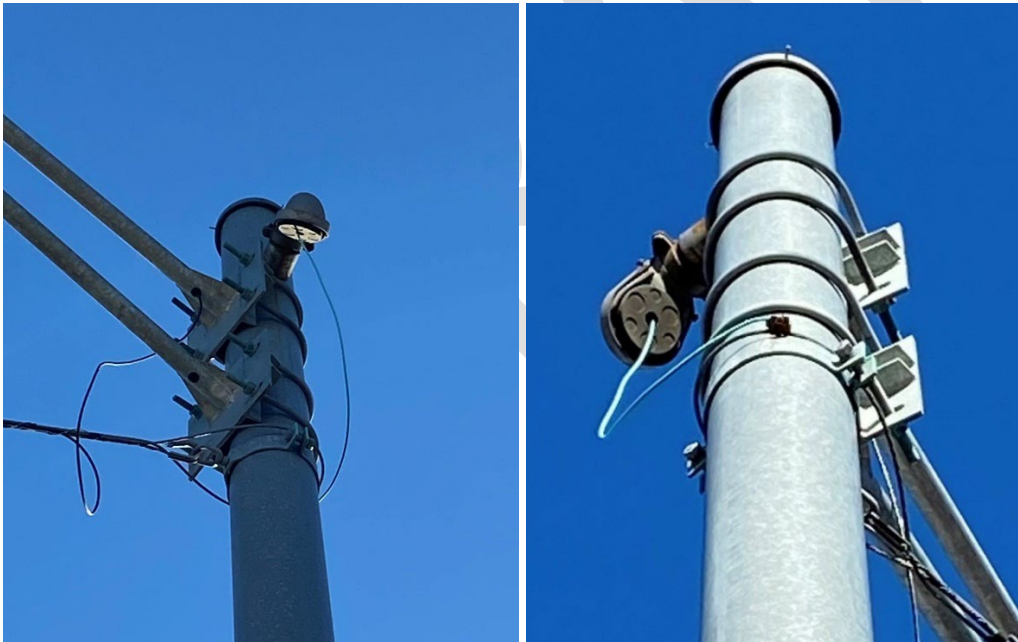
Figure 7-14: Steel strain pole bracket assembly connections for luminaire arms
