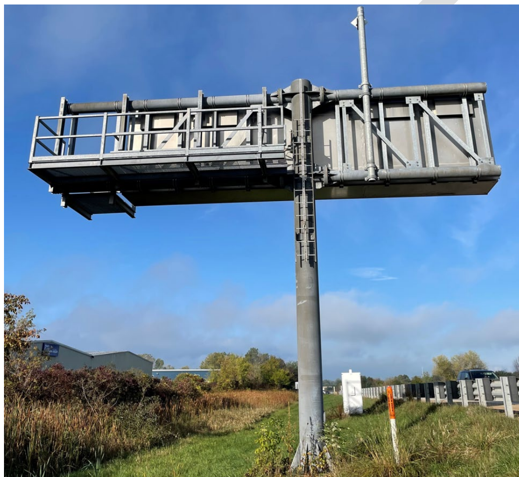
Figure 8.10.1: Dynamic Message Sign Support Structure
