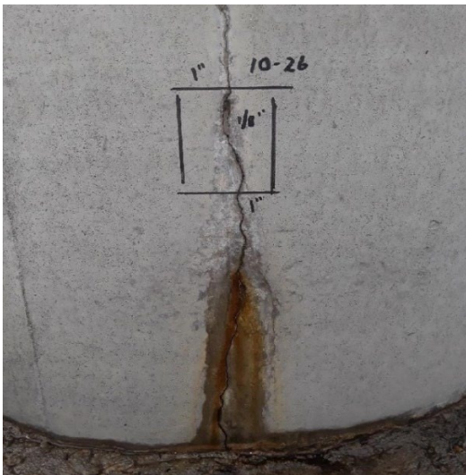
Figure 6-5: Crack with rusted rebar water leakage
