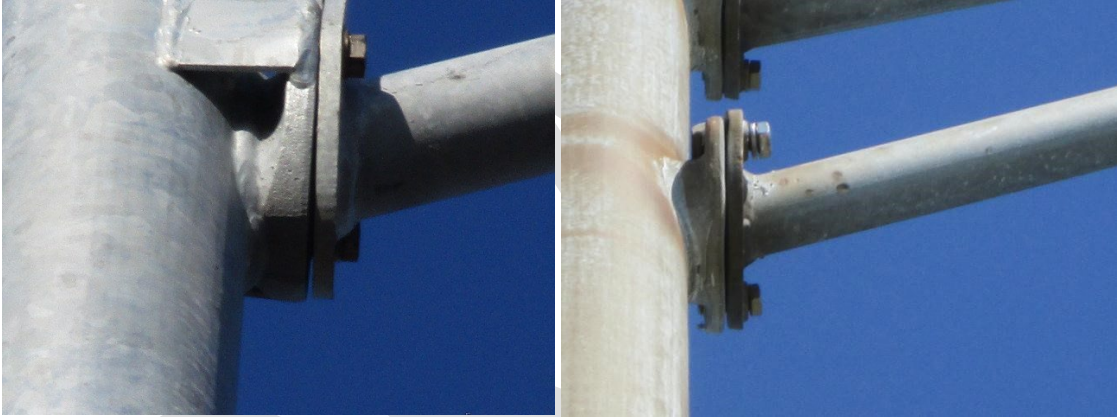
Figure 11-21: Frangible and non-frangible pole structure vertical structure connections, gap at arm flange (left), loose arm connection bolt (right)
