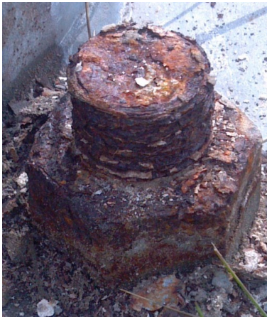
Figure 11-9: Anchor bolt and leveling nuts foundation, non-frangible base anchor bolt corrosion
