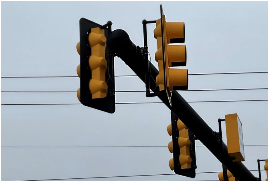
Figure 9-15: Mast arm signal and sign attachment connections
