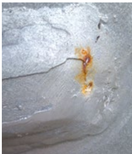
Figure 10-12: Vertical structure connection, rust bleeding through galvanizing at welded gusset plate arm to vertical structure upright
