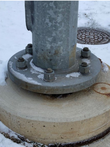
Figure 9-6: Six anchor bolt concrete foundation
