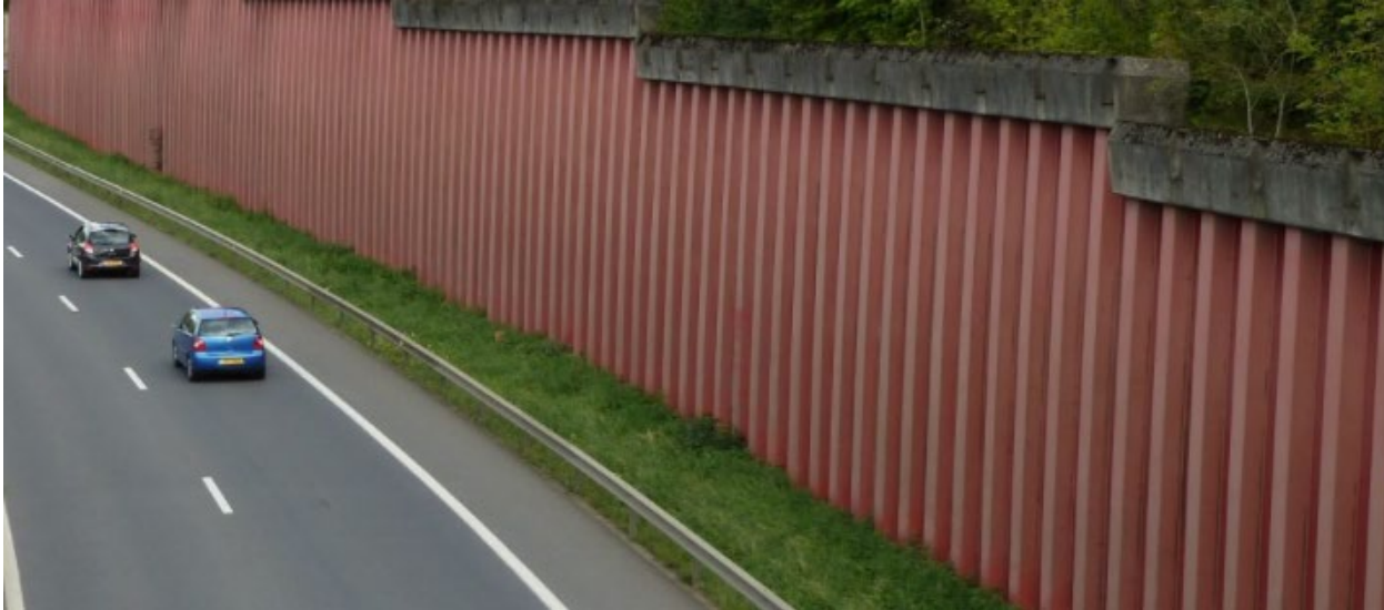
Figure 3-31: Typical continuous wall
