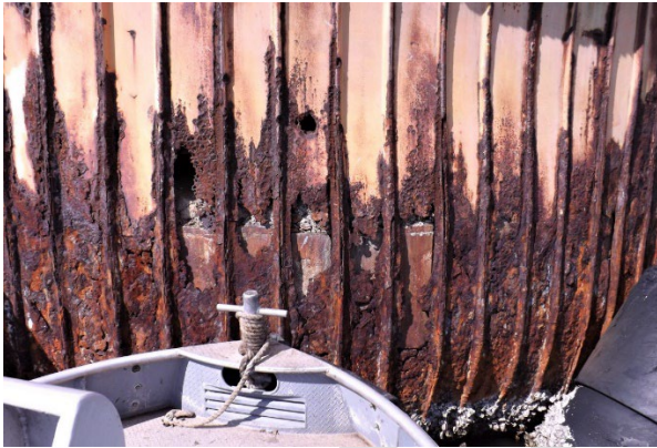
Figure 3-28: Steel corrosion and section loss
