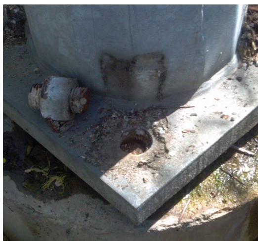
Figure 11-7: Anchor bolt and leveling nuts foundation, severed anchor bolt and nut of non-frangible base
