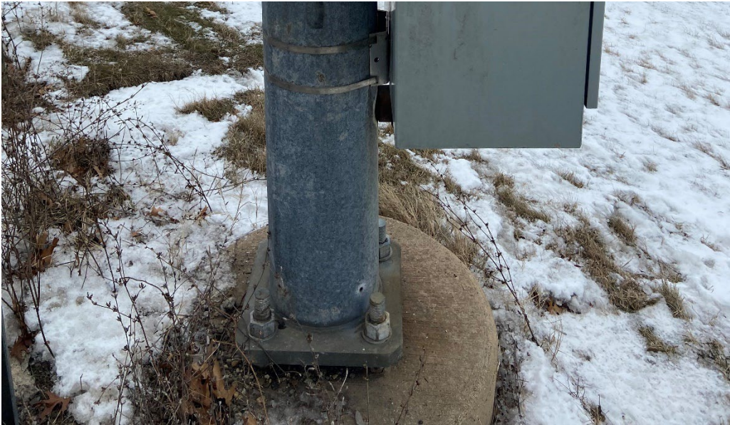
Figure 9-8: Mast arm base plate with four anchor bolts
