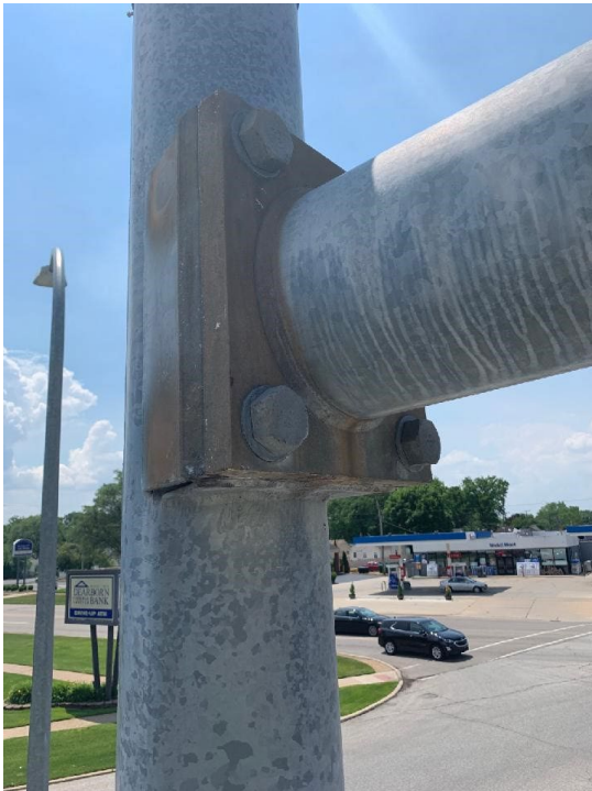
Figure 9-11: Mast arm to pole vertical structure connection, welded box type
