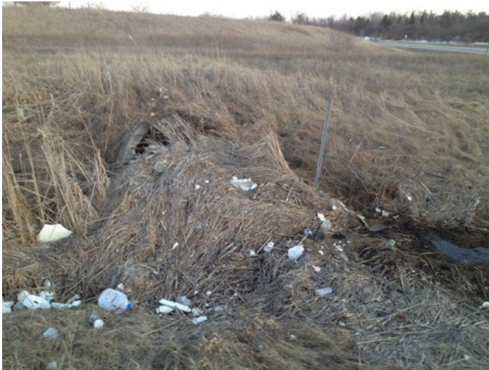
Figure 2-17: Blocked inlet
