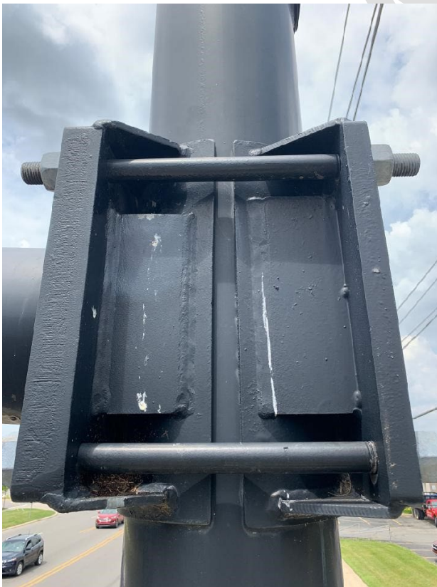
Figure 9-12: Mast arm vertical structure connection, note missing vertical weld on gusset plate
