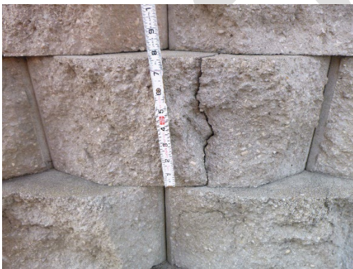
Figure 3-23: Vertical split in modular block
