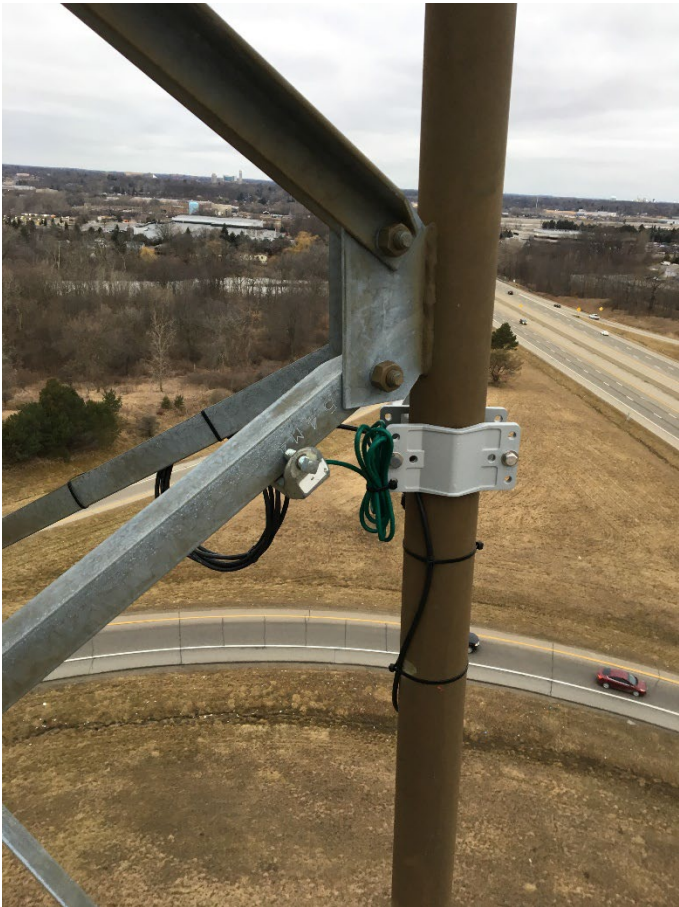
Figure 13-4: Bracing showing vertical structure bolted connection to vertical support
