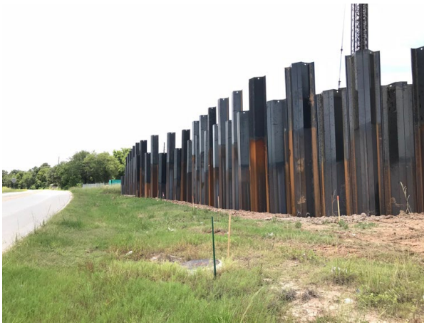
Figure 3-29: Steel protective coating missing
