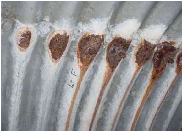
Figure 2-34: Corrosion of a metal culvert
