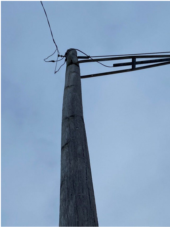
Figure 5-10: Minor crook in wood pole
