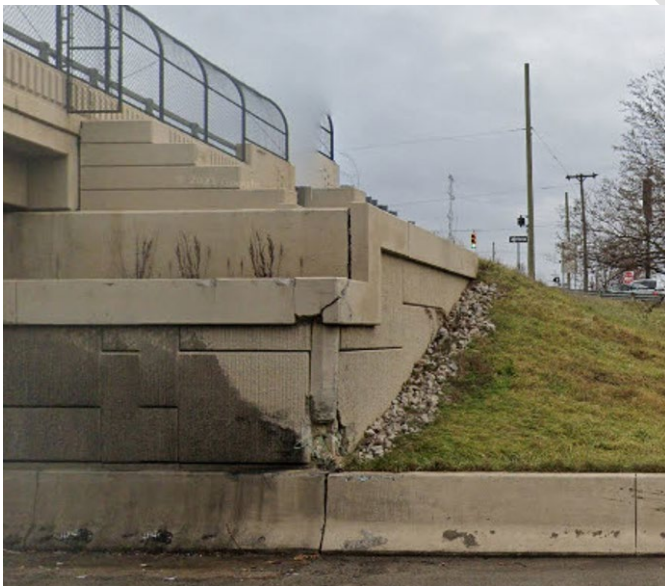
Figure 3-17: Impact damage
