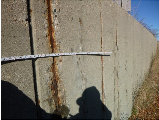
Figure 3-10: Corroded wall reinforcing
