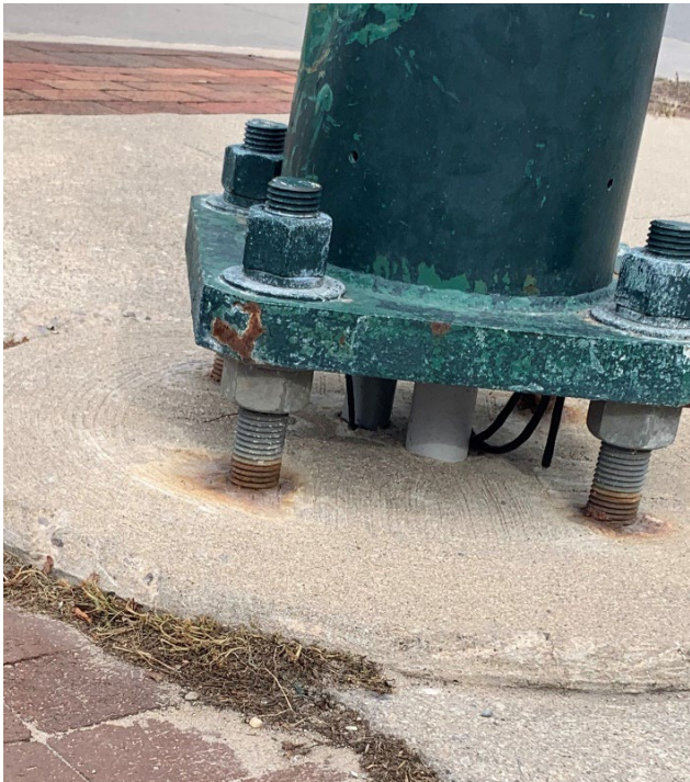
Figure 9-7: Four anchor bolt foundation with excessive standoff distance and corrosion
