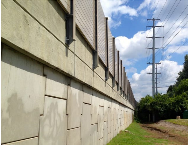
Figure 8-11: Noise wall attached to retaining wall
