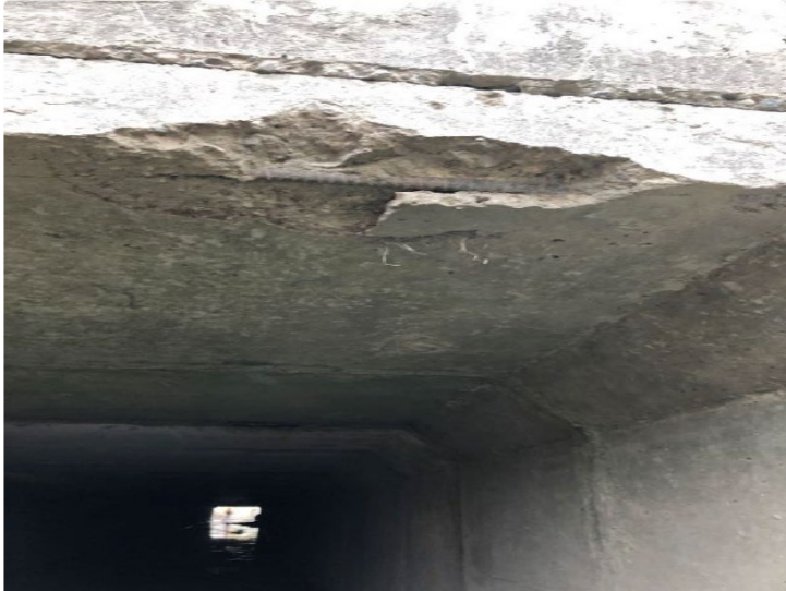
Figure 2-25: Spalled concrete at headwall
