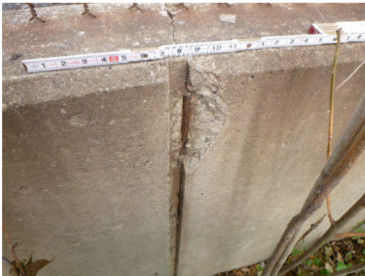
Figure 3-11: Concrete spall with corroded reinforcing
