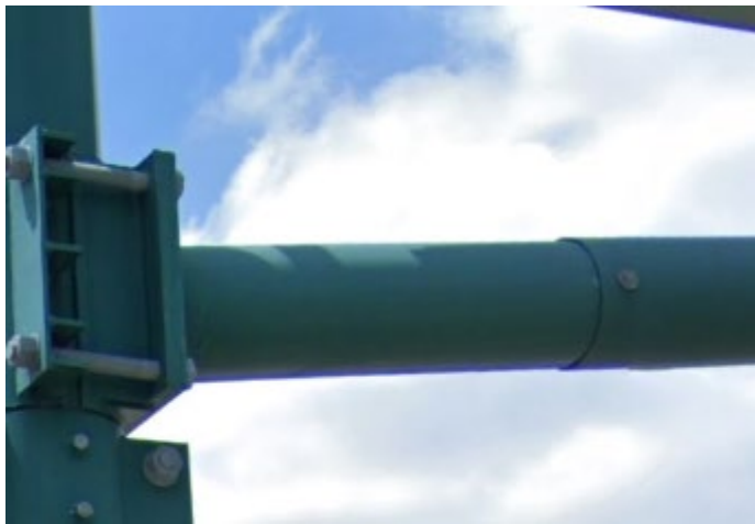
Figure 9-14: Mast arm member splice with connection bolt
