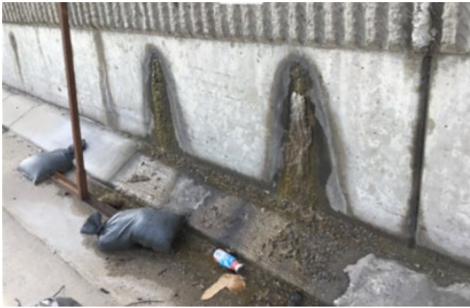
Figure 3-16: Weep holes/wall drainage
