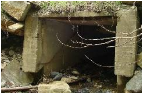
Figure 2-14: Vertical alignment issue leading to foundation undermining
