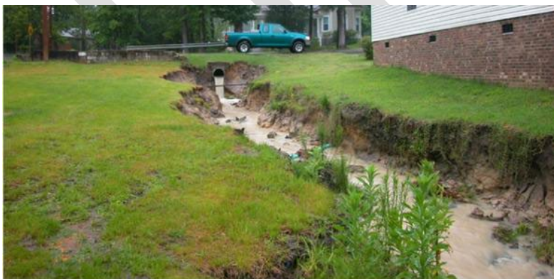
Figure 2-19: Bank erosion
