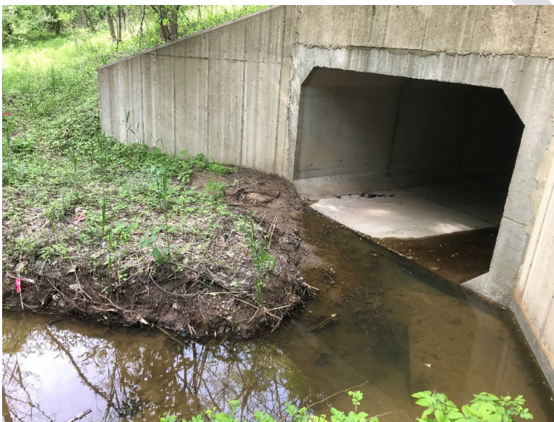
Figure 2-13: Stream channel poor horizontal alignment
