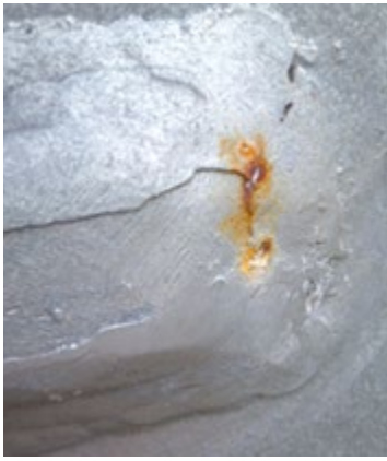
Figure 4-14: Vertical structure connection, rust bleeding through galvanizing at welded gusset plate arm to vertical structure upright
