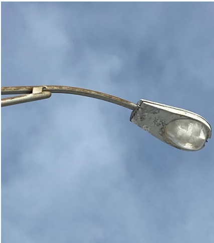
Figure 11-22: Luminaire and luminaire arm element, evidence of galvanizing damage
