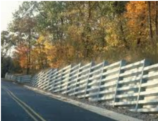
Figure 3-27: Typical metal bin wall
