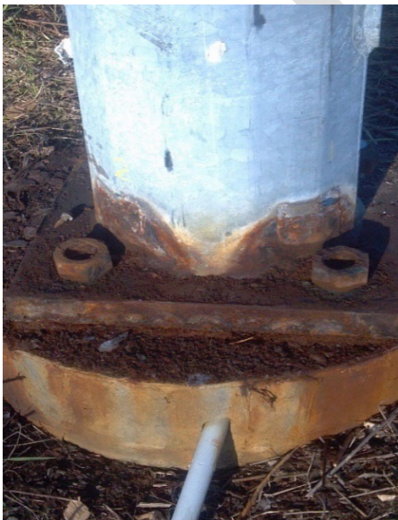
Figure 11-15: Non-frangible pole structure base plate, corrosion of base plate, anchor bolts, and nuts and inadequate bolt projection
