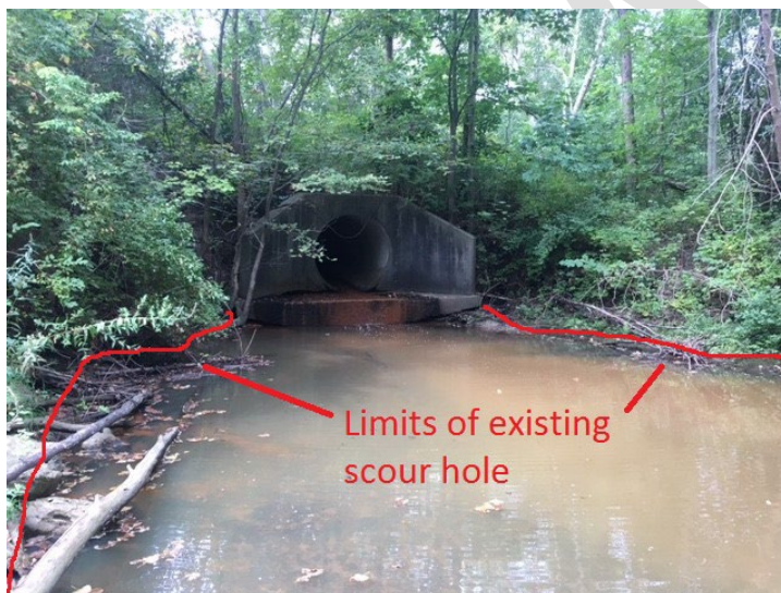
Figure 2-27: Perched outlet with large scour hole
