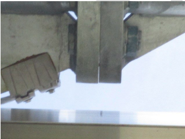
Figure 10-13: Horizontal structure connection, gap between arm connection flanges
