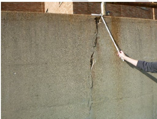
Figure 3-12: Spalled and delaminated concrete
