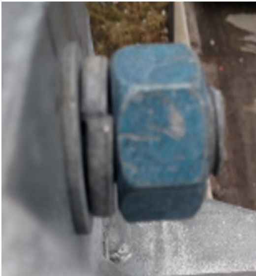
Figure 4-13: Vertical structure connection, loose bolt/lock washer not fully compressed
