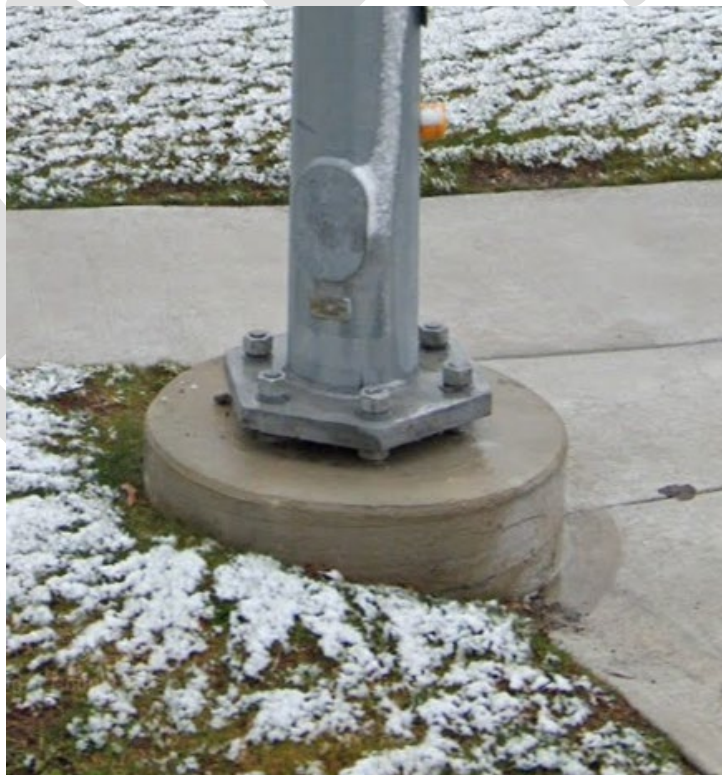
Figure 7-6: Steel strain pole (multi-sided) structure with four anchor bolts (left) and six anchor bolts (right)
