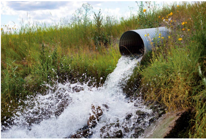
Figure 2-21: Projecting or perched outlet
