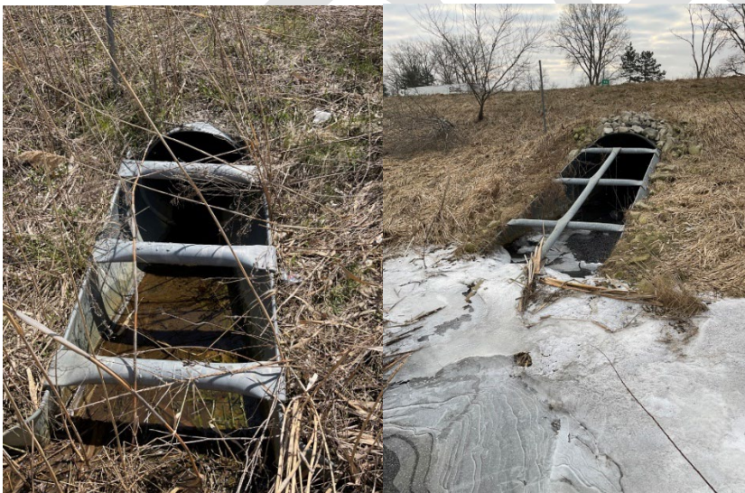
Figure 2-22: Sloped metal end sections
