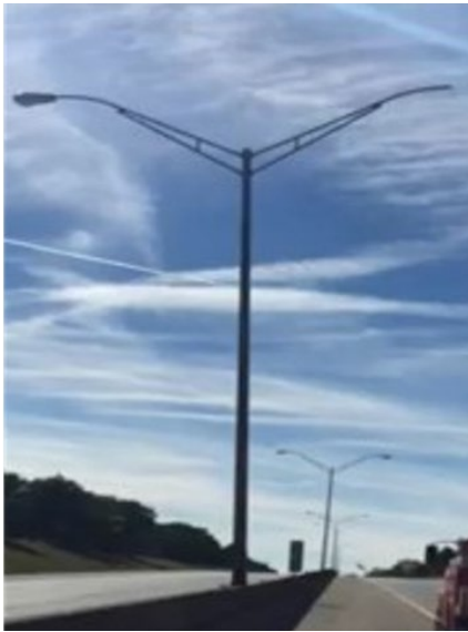
Figure 11-23: Luminaire and luminaire arm element, missing luminaire head
