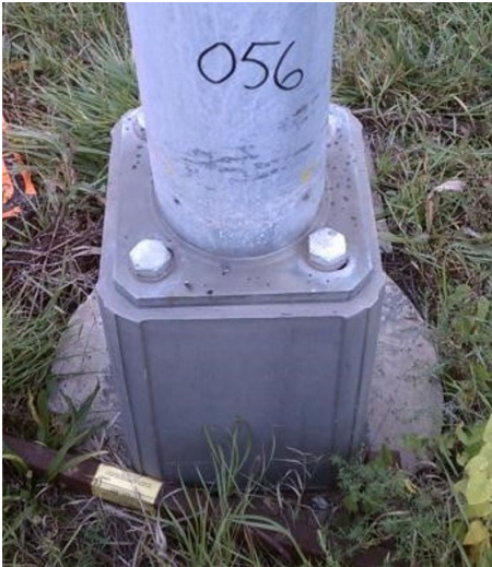
Figure 11-13: Frangible base connections, exposed bolt hole
