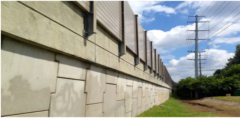
Figure 8-5: Noise wall attached to retaining wall
