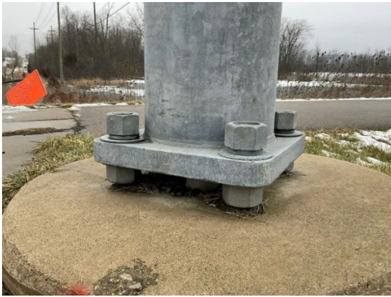
Figure 7-9: Anchor bolt negative projection – the top of the anchor bolt is not flush or higher than the top of the nut
