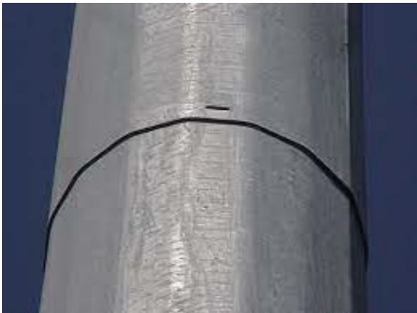
Figure 12-6: HMLT pole splice
