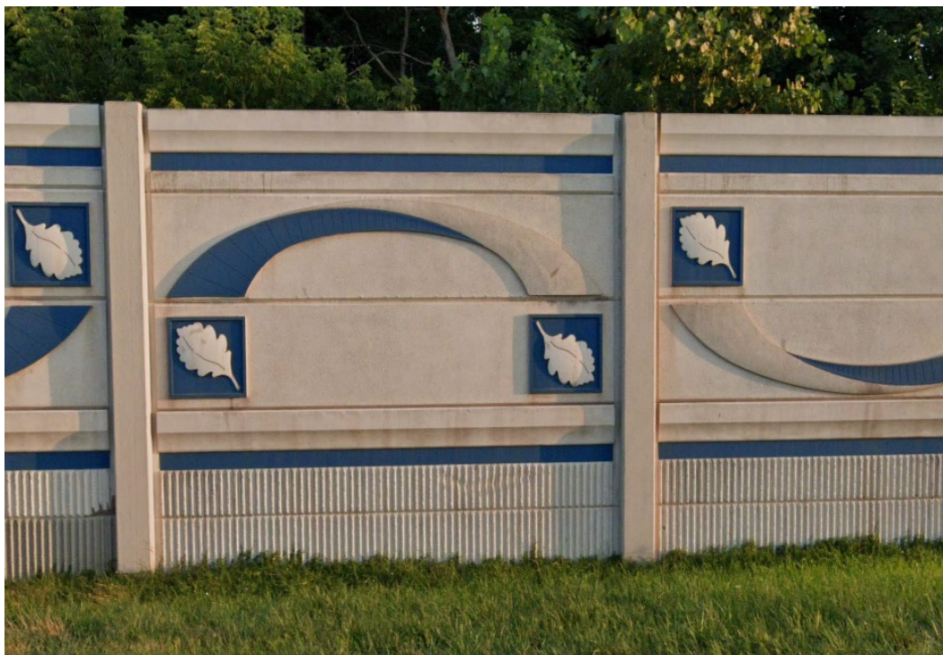
Figure 8-7: Noise wall with architectural features with vertical supports and horizontal members
