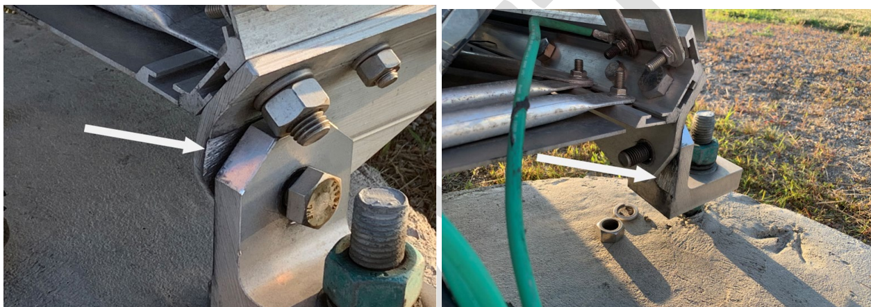
Figure 14-8: Evidence of wear on metal due to oscillation along with loose connection
