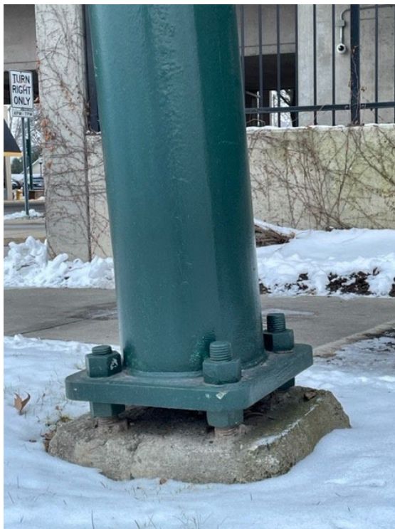
Figure 7-7: Steel strain pole square foundation with four anchor bolts (left, note misalignment), newer style drilled shaft foundation with six anchor bolts (right)
