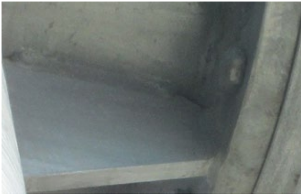
Figure 4-12: Vertical structure connection, missing flat washer on head side of bolt
