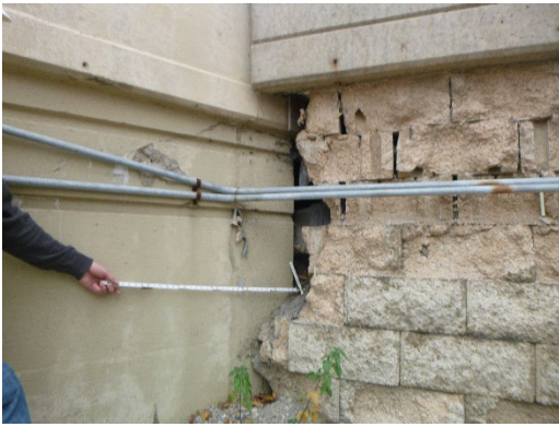
Figure 3-24: Masonry breakdown
