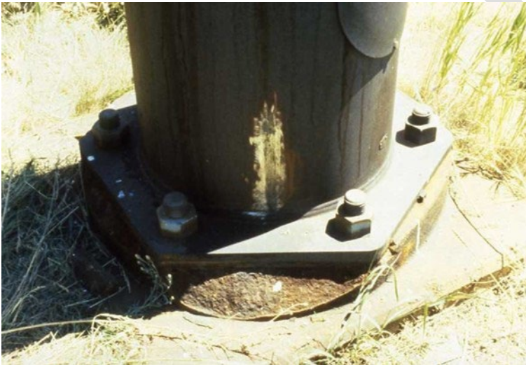
Figure 12-4: HMLT concrete foundation, spalling deterioration
