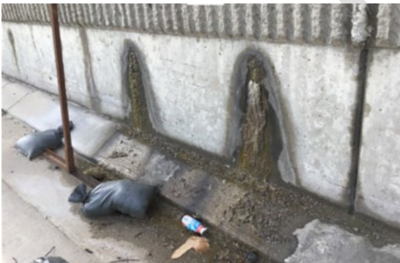
Figure 3-13: Retaining wall concrete abrasion
