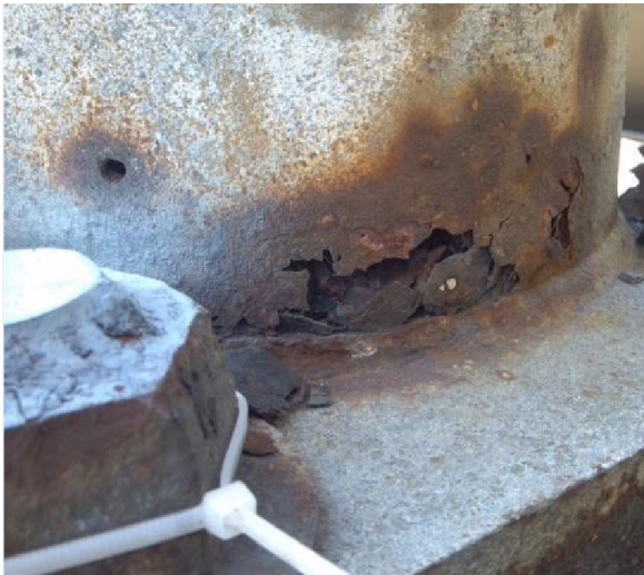
Figure 11-16: Base plate, pole corrosion and section loss at base weld
