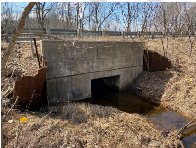
Figure 2-24: Concrete headwall and metal sheet pile wingwalls
