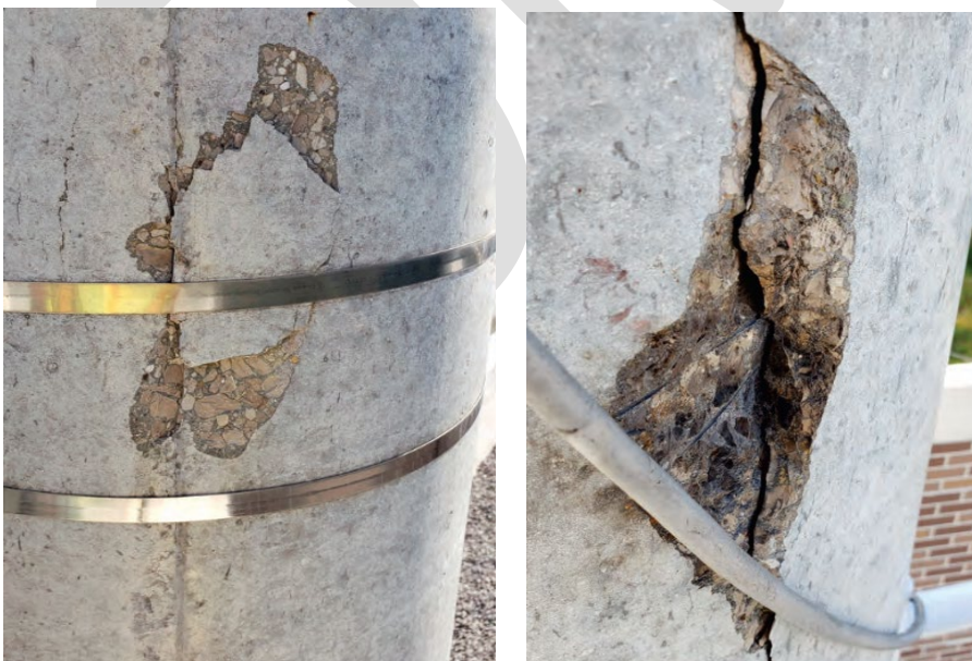
Figure 6-6: Spalls (left), major cracking and spalls (right)
