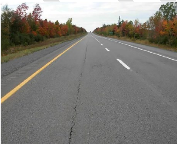
Figure 2-6: Longitudinal cracking
