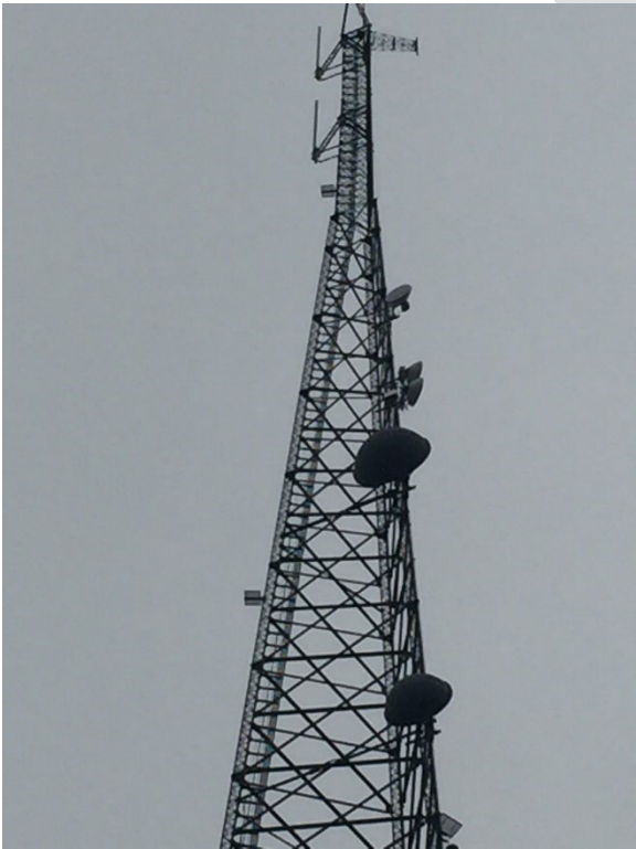
Figure 13-3: Communication tower with vertical supports and diagonal and horizontal bracing
