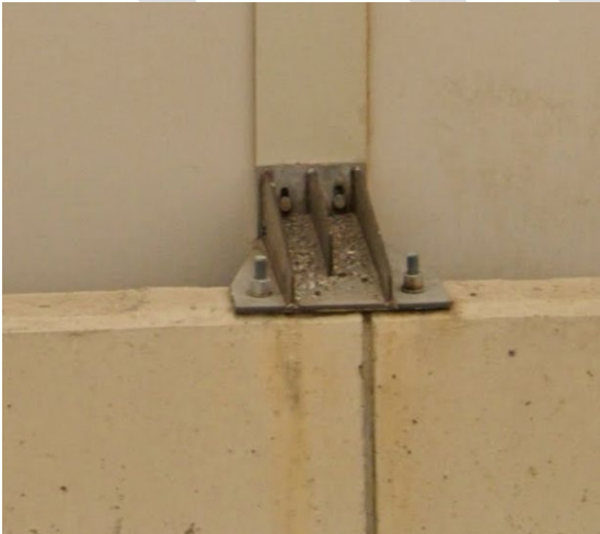
Figure 8-10: Noise wall attachment to concrete barrier
