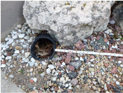
Figure 3-43: Drainage outlet is partially clogged with leaves and debris
