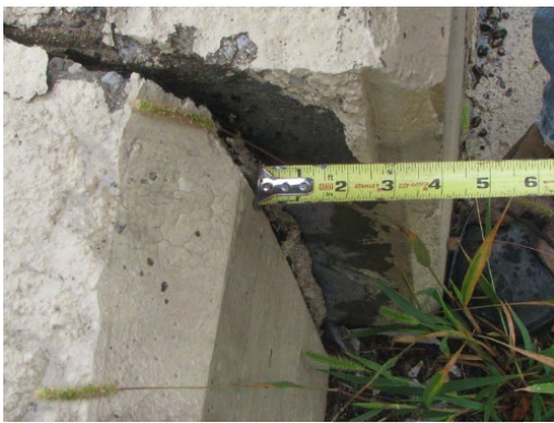
Figure 3-36: Wall displacement
