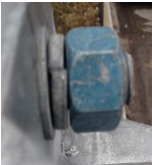
Figure 10-11: Vertical structure connection, loose bolt/lock washer not fully compressed
