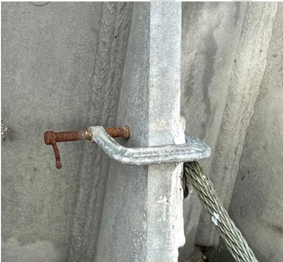
Figure 10-8: Corrosion in bonding clamp along bolt of base plate stiffener
