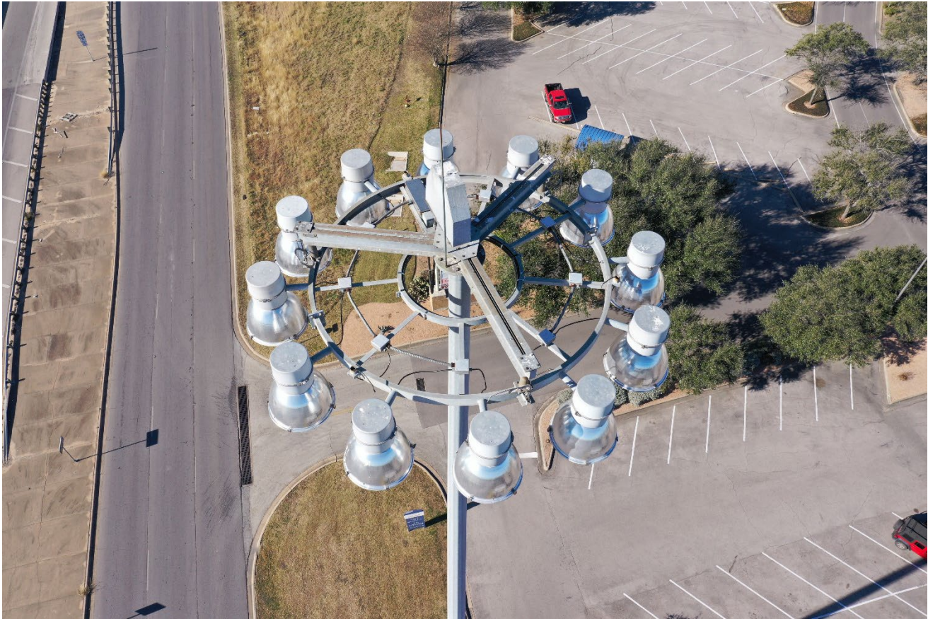
Figure 12-3: High-Mast Lighting Tower, aerial view of tower and lighting array from UAS
