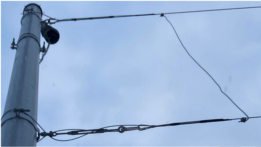
Figure 7-16: Span wire assemblies attached to steel strain pole band clamps
