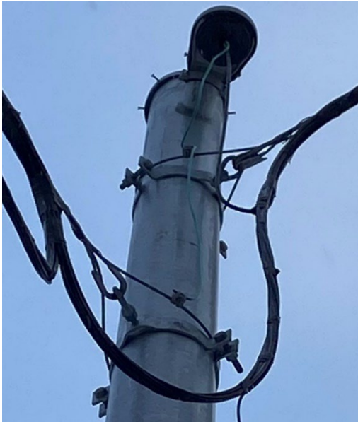
Figure 7-13: Steel strain pole band clamp connections for span wires
