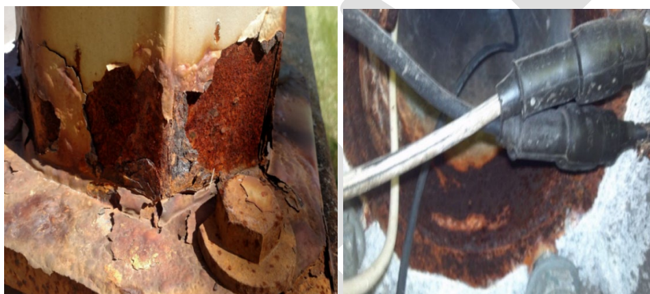
Figure 11-17: Non-frangible pole structure vertical support column (upright), coating system failure and corrosion in upright at base weld (left), corrosion inside column (right)
